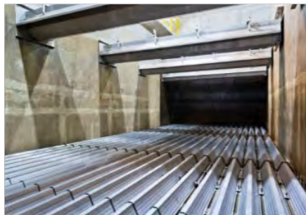
Phoenix Underdrain System
